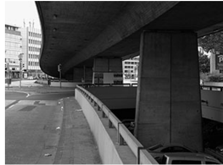
Arne Schmitt, from Bunkererfahrung / Bunker Experience , 2013
